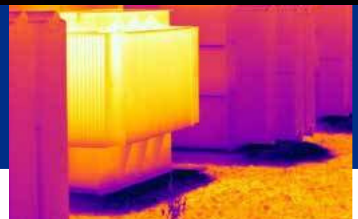
Transformer Thermal Image
