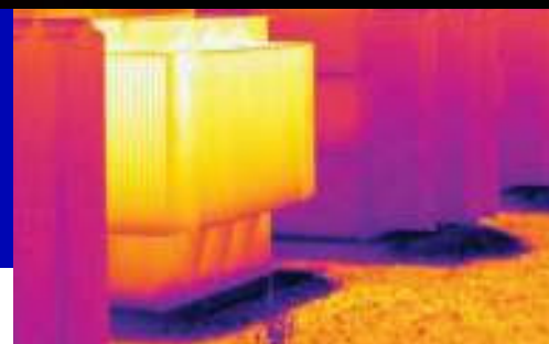
Transformer Thermal Image
